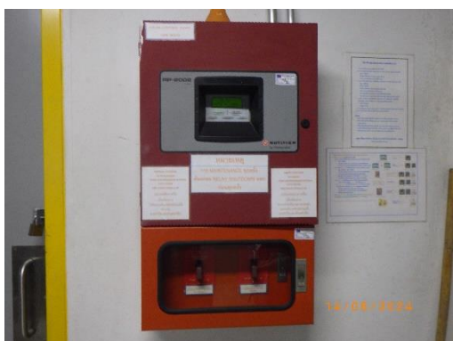
Fire Alarm Control Panel
